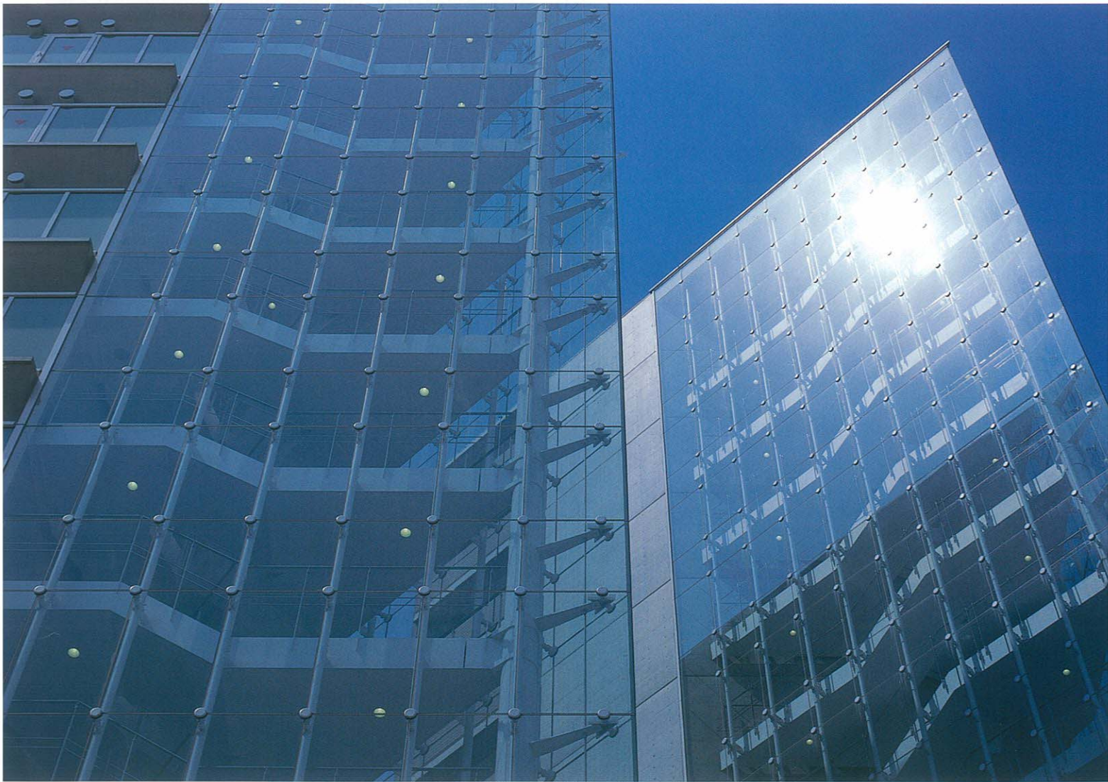
A棟、B棟階段 Stairs, Residence Hall A and B
